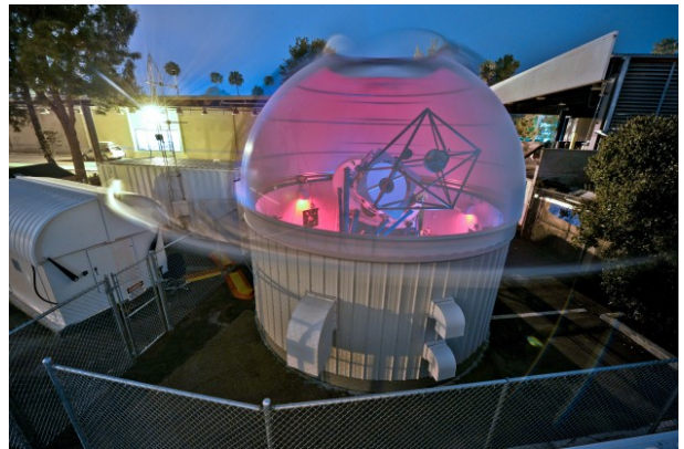
Long exposure of a LCOGT 1m as the dome rotated, showing site services container with weather tower.
